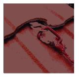
Install an anchor above the area being built: Choose an anchor that is appropriate for the tile type and anchor location. Depending on the roof design, the best location might be at the peak of the roof, directly over a truss.
